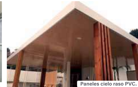
Paneles cielo raso PVC.
